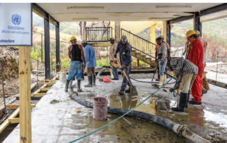
Workers completing the foundation for the Salisbury Educational Facility in Dominica
