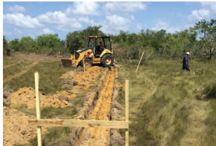
Construction of a fence for the Belize Youth Challenge Compound
