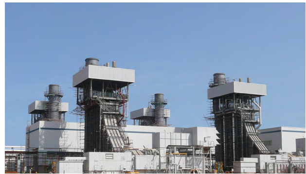
Exterior view of power island of Ghana power plant (2 gas turbines + 4 boilers + 4 gas engines)
