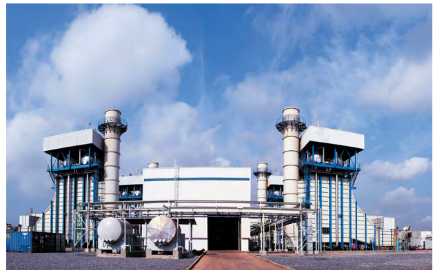
Panorama of Ghana power plant
