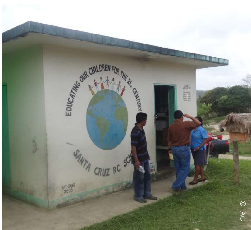
Old kitchen and storage room, July 2016.
