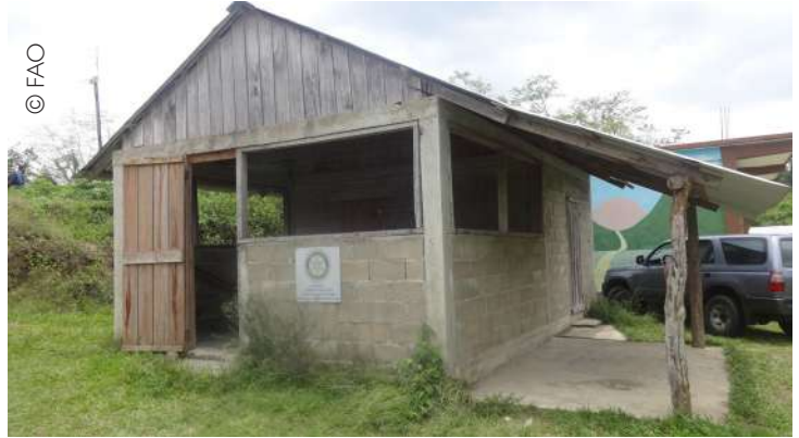
Old kitchen infrastructure, July 2016.
