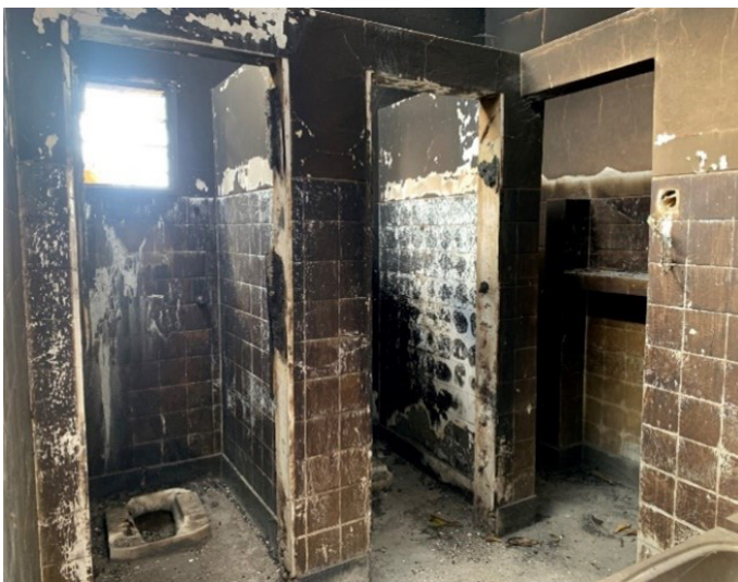
Before and after the Health Centre's refurbishment
