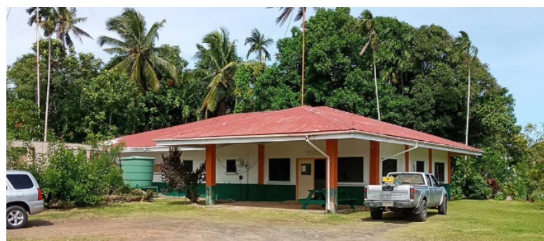
Northern Community Health Clinic during rehabilitation
