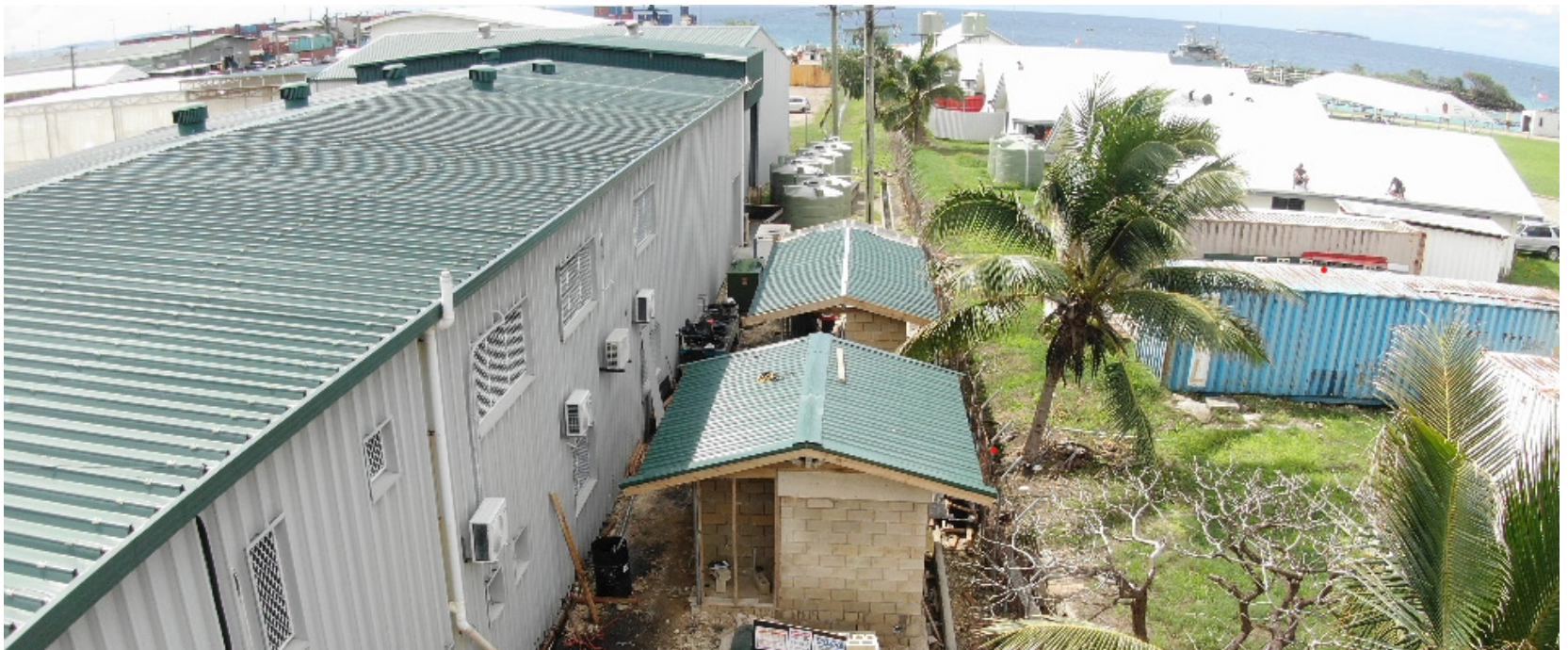
Construction of Tonga's new Food Processing and Export Building
