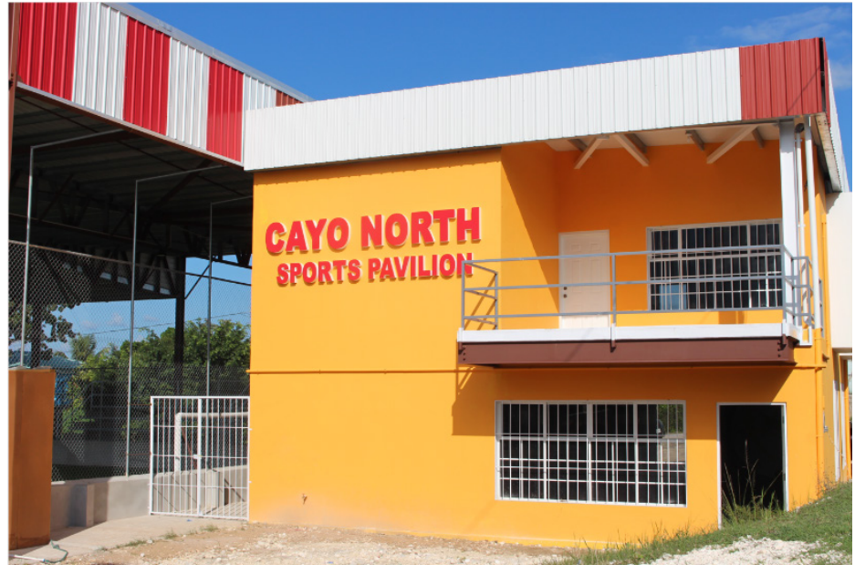
Cayo North facility
