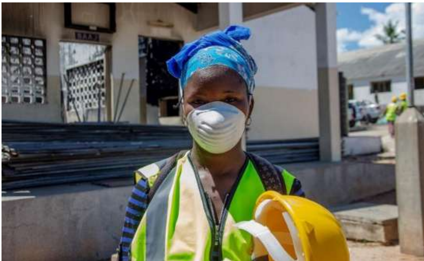
Ms. Mendonca Joao, during refurbishment work
