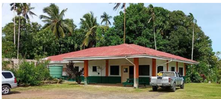
Northern Community Health Clinic during rehabilitation
