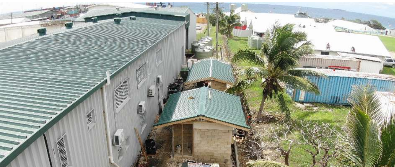
Construction of Tonga's new Food Processing and Export Building
