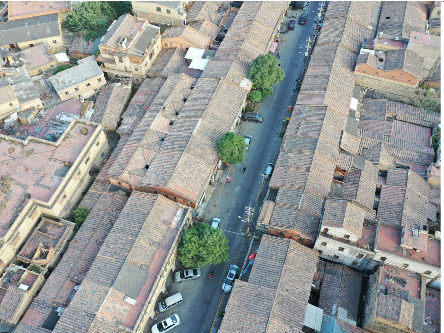
5. Aerial view of arcaded buildings
