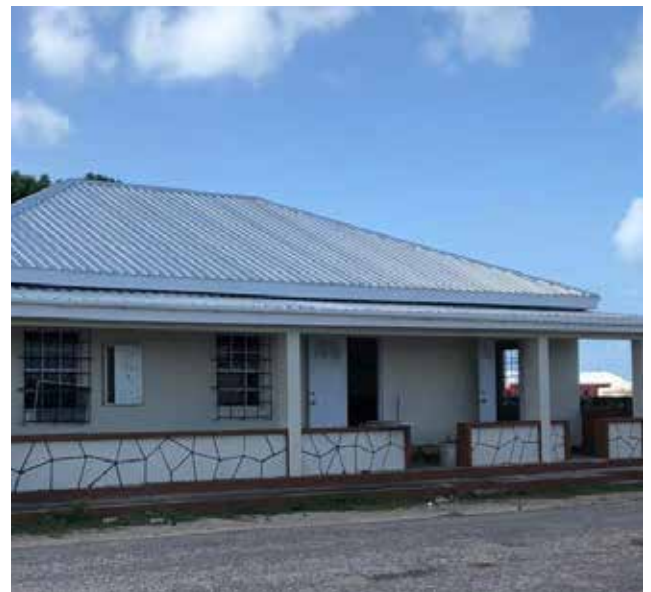
POST OFFICE AFTER REHABILITATION
