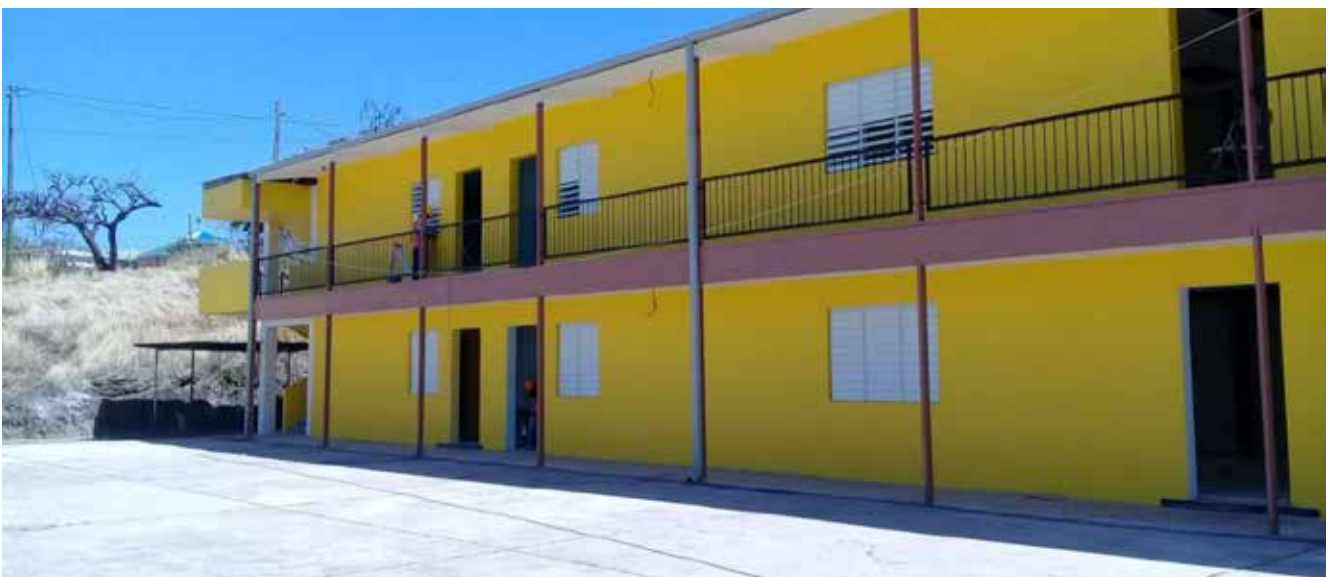
SALISBURY SCHOOL COMPLEX AFTER RECONSTRUCTION
