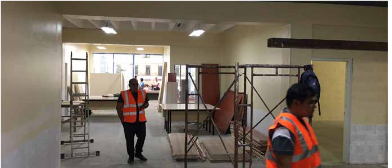
BEFORE AND DURING THE REFURBISHMENT
