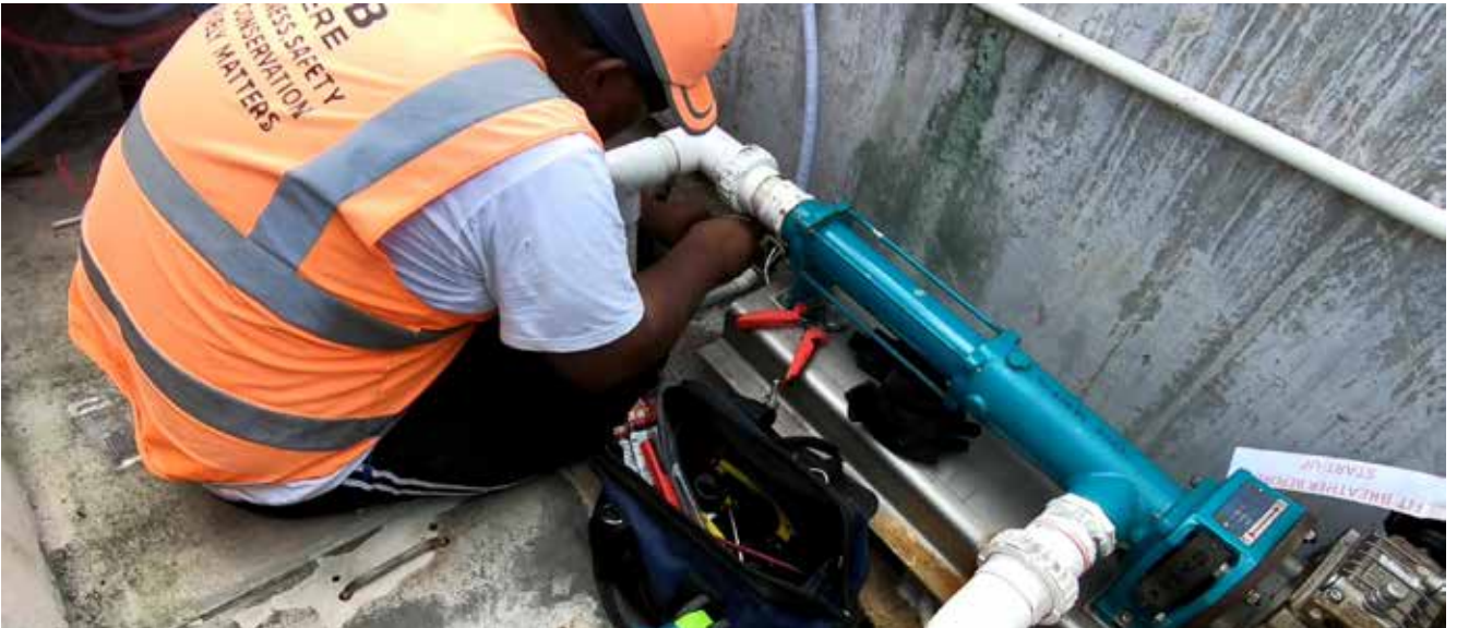
AT WORK DURING BONRIKI SALINITY METRE INSTALLATION AND TESTING
