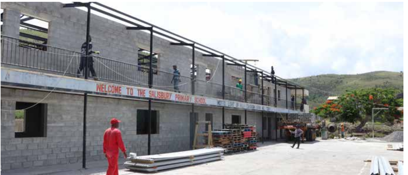
SALISBURY SCHOOL COMPLEX DURING RECONSTRUCTION
