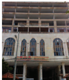
Before the rehabilitation
