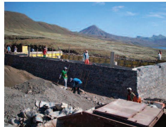
Building the reservoir
