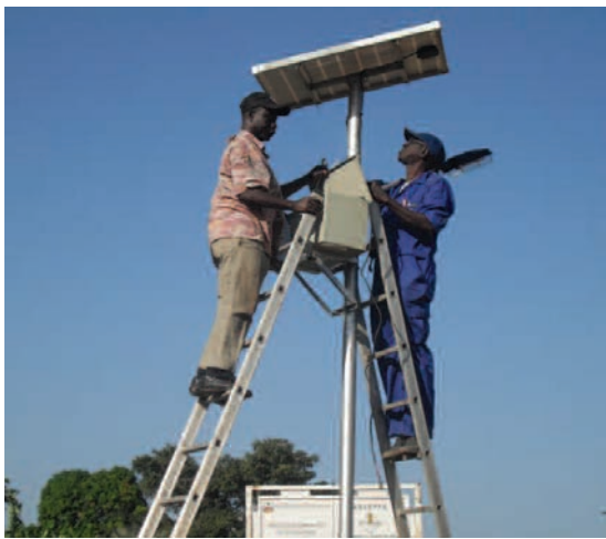
Technicians install solar panels
