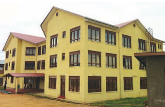
Reproductive health centre built by the project
