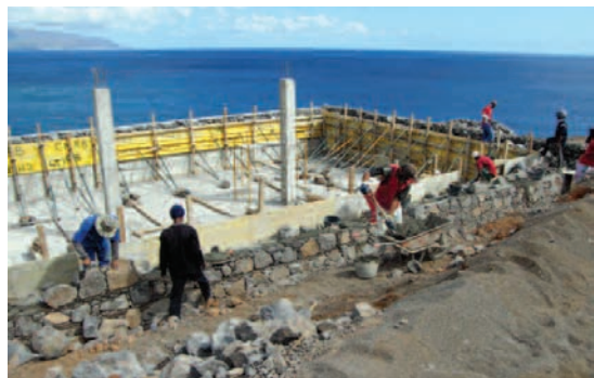
Building the reservoir
