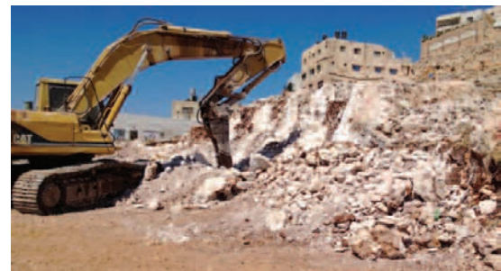
Excavation works in Nablus
