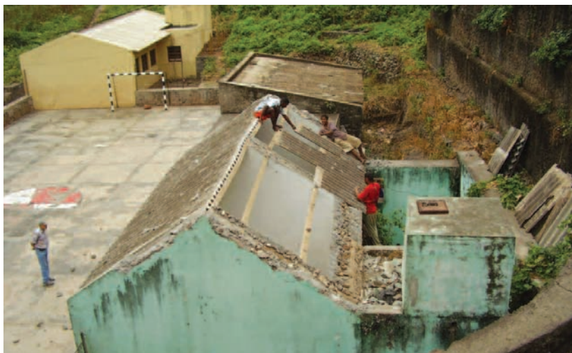
Dilapidated health-care centre before refurbishment
