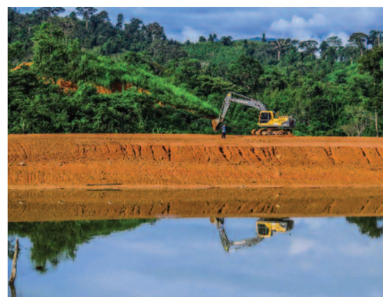
Repairing the irrigation scheme in Nam Phou, Bolikhamxay Province
