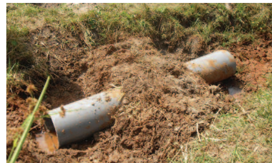
Rehabilitation of low-lying rice fields with PVC tubes
