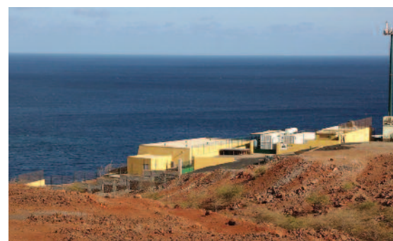
Water desalination plant at work
