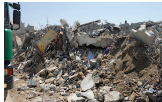
Project site before reconstruction of the Hospital
