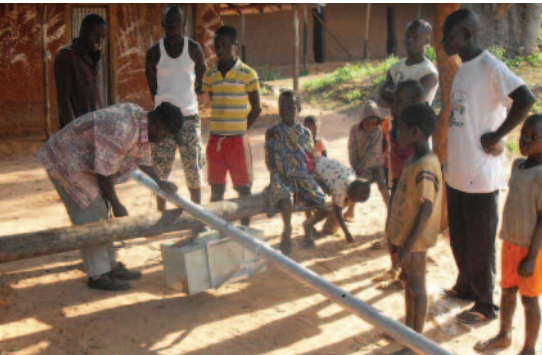
Preparations to install a street light
