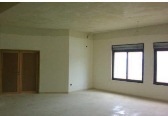
Progress on the building's interior
