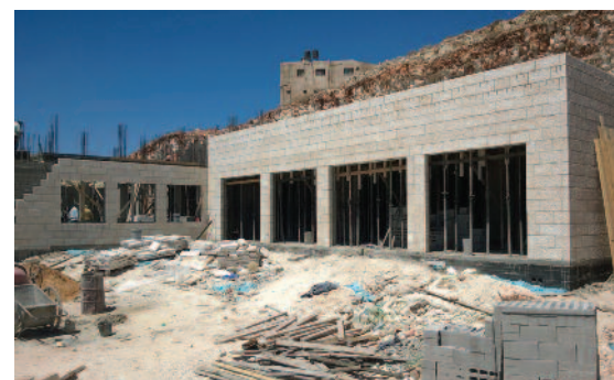
Ongoing construction at the project site
