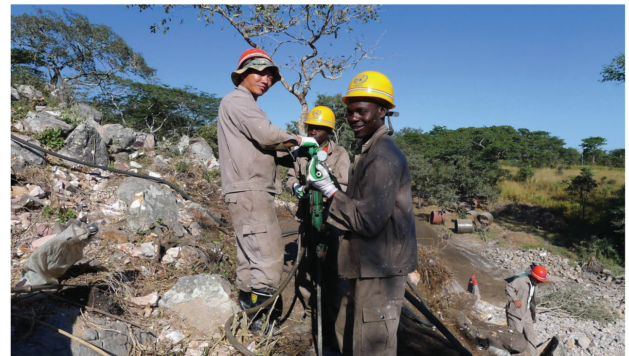
Shiwang'andu Small Hydro Power Project
